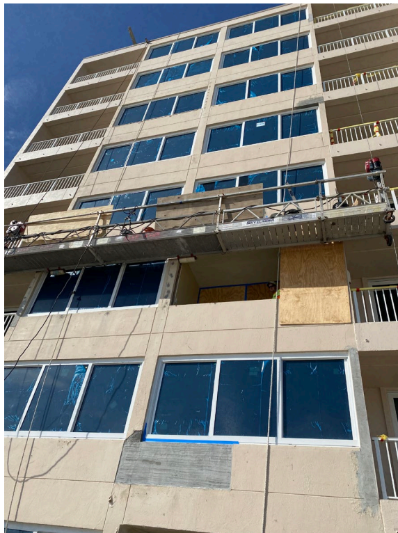
Picture 6: In-progress work on the 10/11 stack
