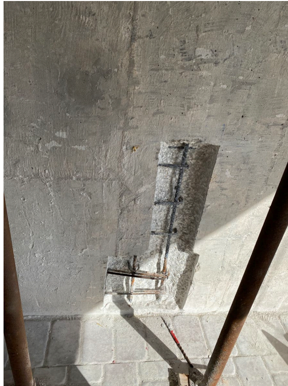
Picture 1: Typical wall repair
