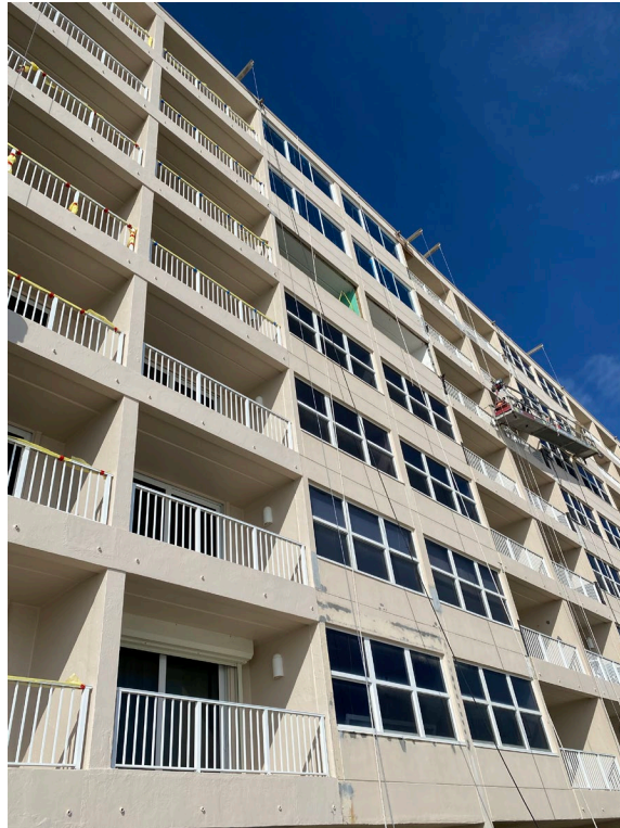
Picture 5: In-progress work on the 08/09 stack
