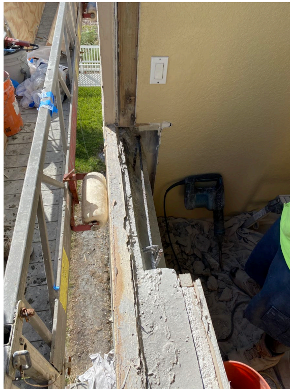
Picture 2: In-progress concrete repair at Unit 210 window sill
